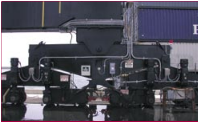
Figure 5. Crane gantry after refurbishment.
